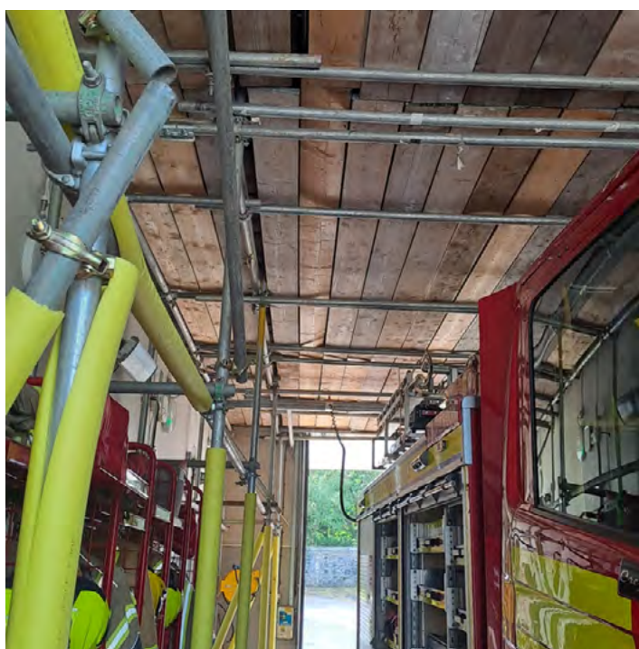
Image 1: Stewarton Fire Station, Appliance Bay
